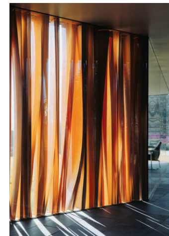
Holzurniere in der Fassade Private Bibliothek, Laufen Wood veneer in the façade Private library, Laufen
