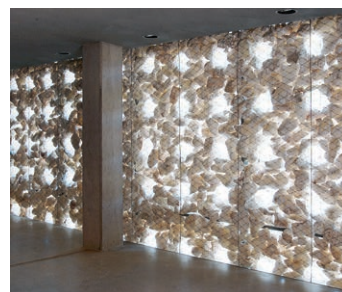
Alabastersteine in der Fassade Ausbau Alpinarium, Galtür Alabaster stones in the façade Alpinarium extension, Galtür
