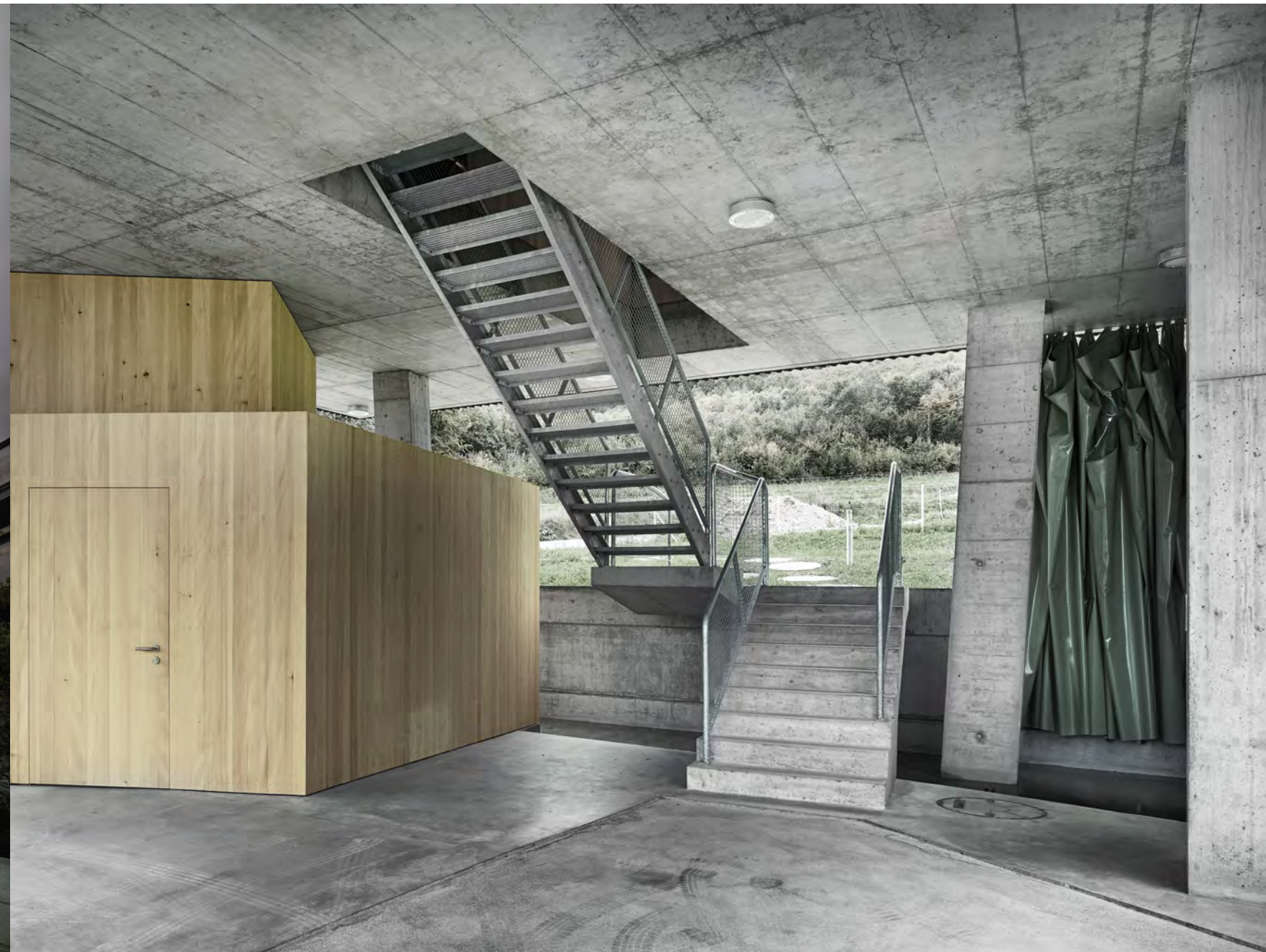
The landing of the open staircase leads to the front door on the first floor.
