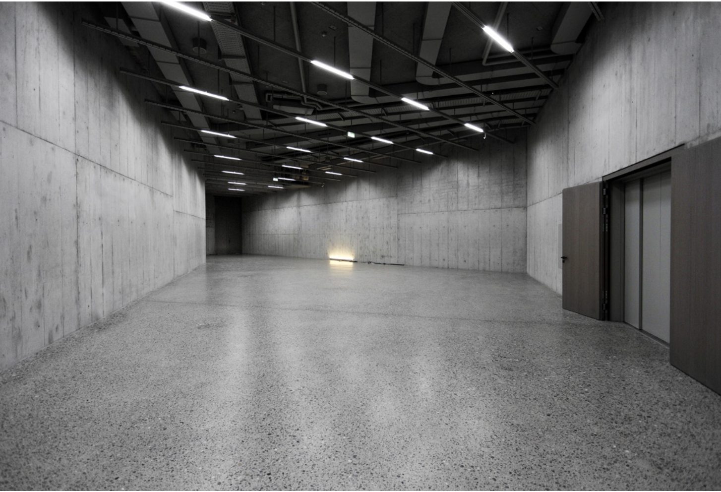
The interior of the new building is executed in exposed concrete.
